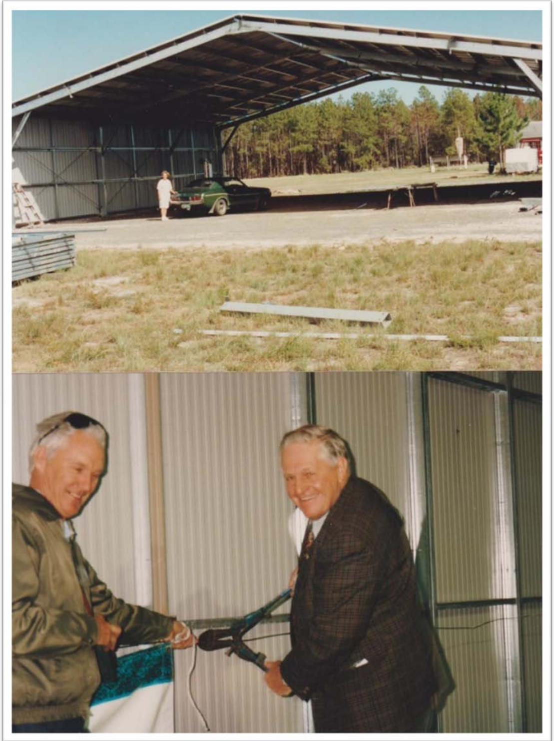
Hangar under construction and being opened by Bill Neubecker.
